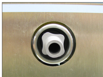
Installed Drain Fitting with Cap Removed
