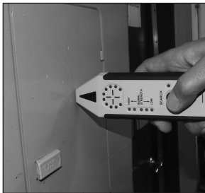
Finding Breaker Panel
