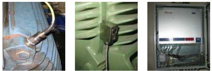
Range of SKF sensors monitoring defined points and SKF IMx online surveillance system
