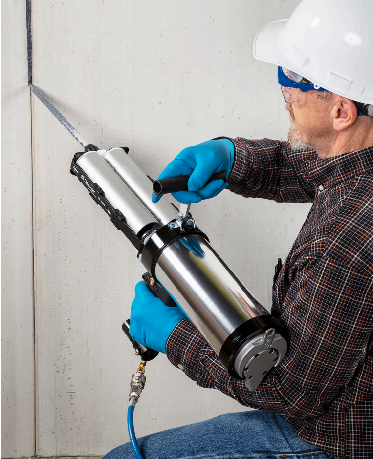
Powerful 2K pneumatic dispense guns are ideal for crack injection applications.
