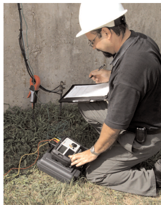
Using ART method with the DET3TC to test commercial ground without disconnecting the system
