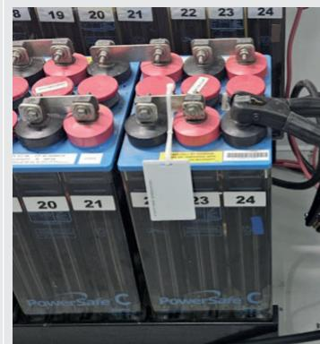
The RFID tag number will now show up on the configuration screen. Now when this tag is scanned this battery string configuration will be called.
