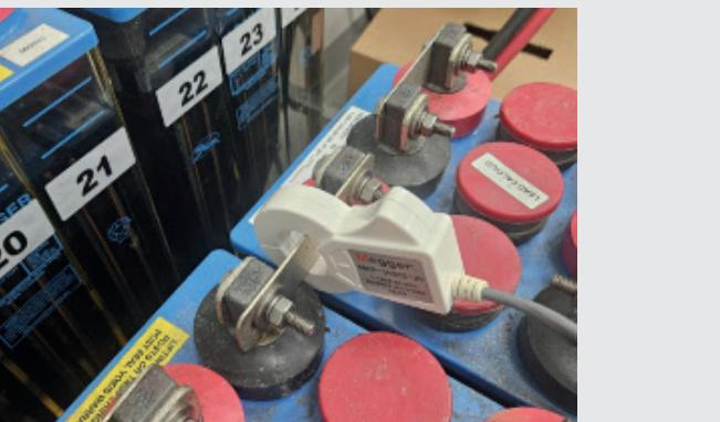
Continue taking measurements of each cell and strap in sequence until you reach the last cell in the string. When the BITE5 ADVANCED measures the last cell in the string, it will display a summary.
