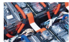
Connection resistance of battery busbars
