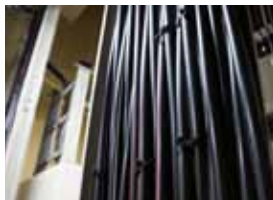
Locations without energized parts
