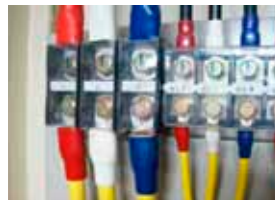
Locations with covered terminals
