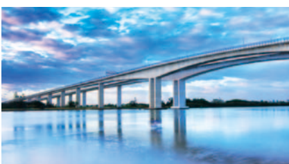
Monitor infrastructural deterioration in bridges
