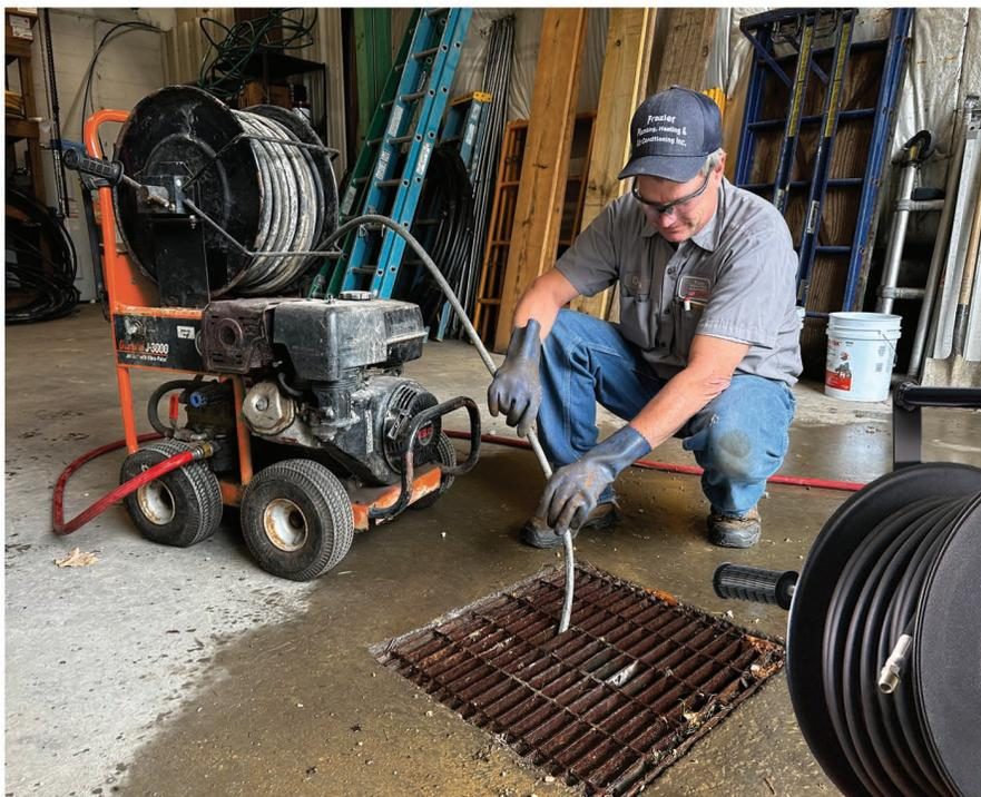
“What’s nice about it is it pulls through sewer lines full of debris. We thought we had a leaf blockage in an outside drain line, but when the jet punched through it, we found the line was packed with acorns, sand, and mud. We even blew shale out of the line”
