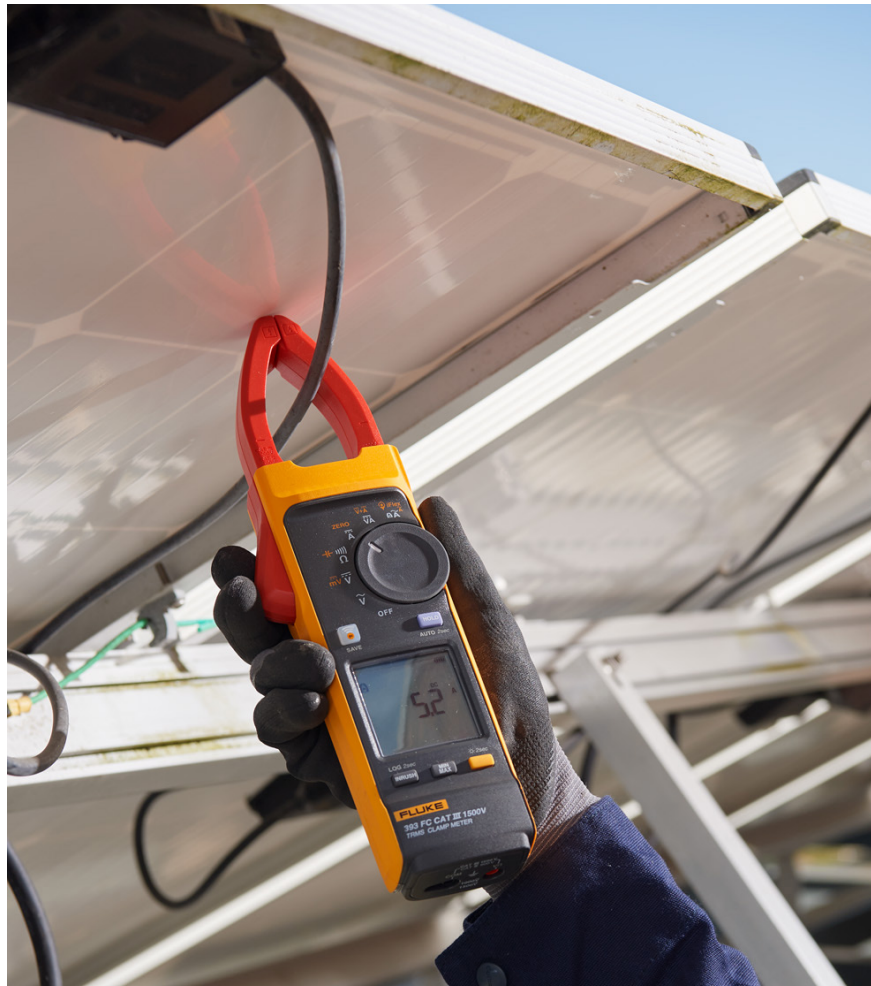
Measuring current on a PV panel with a Fluke 393 FC clamp meter.
