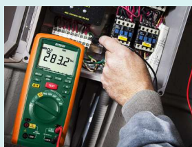
Voltage check on motor starter
