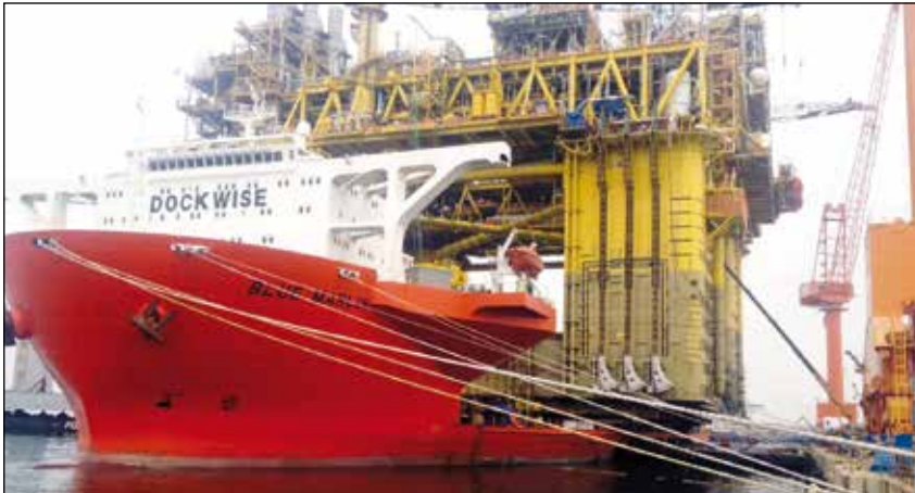
▲ The superlifting and launch of a 43.000-ton floating oil production system in Malaysia for the Gumusut-Kakap offshore field has set high benchmarks for safety through its use of sophisticated EVO-Series synchronous hydraulics to lift, balance, weigh and smoothly launch massive resources structures.
