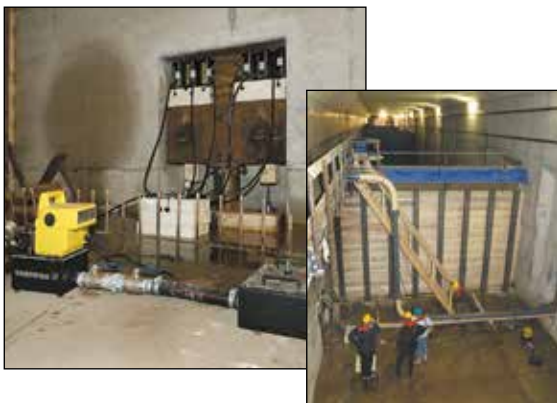
◀ The unique Enerpac RA-Series cylinders – lightweight and made of aluminium alloy – these RAC-506 cylinders are ideal for the positioning of tunnel elements under the river. (High Speed Train Line, The Netherlands)
