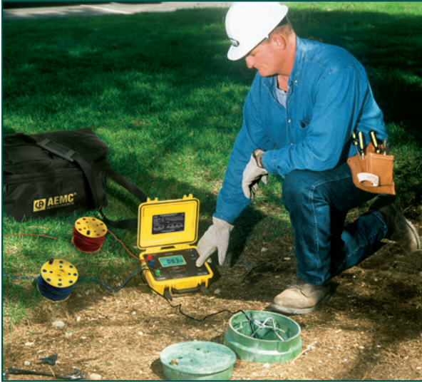
Model 4630 performing a 3-Point ground resistance test on an individual rod.
