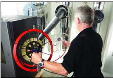
Fig. 20: Cleaning a stainless steel chimney
