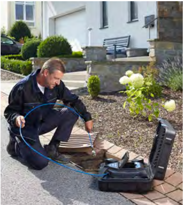
The 100' push rod and the pan- and tiltable camera head 1.5" make sure nothing in the house supply line remains hidden from your view.
