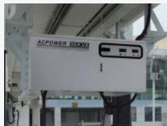
Airport Apron / Hangar
