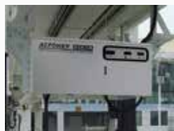
Airport Apron / Hangar
