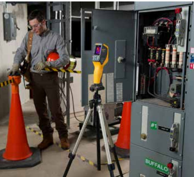
Automated monitoring alarms available on the VT04.
