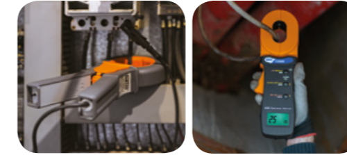
Measurement of leakage current with optional clamp HT96U.
