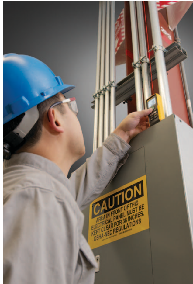
Measuring height to tall ceiling.
