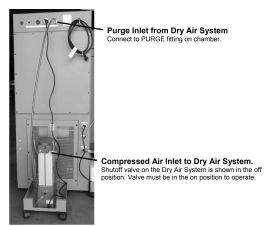
Figure 4.4 – Dry Air Purge System Installation
