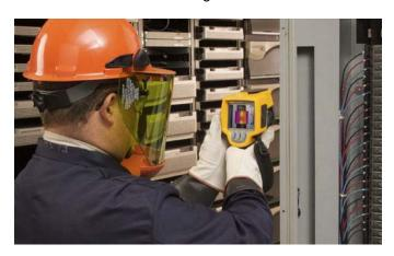
Abnormally hot electrical connections are not only a potential early warning of failure and a safety hazard, they're also consuming excess energy.
