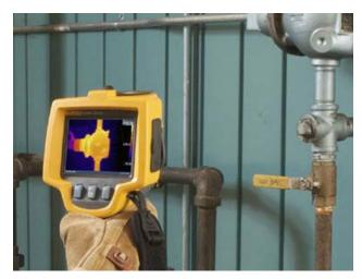
If your facility uses a boiler, scan the steam lines to check for leaks, blockages, and failed traps.
