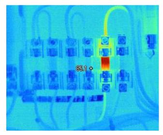
When evaluating an electrical hot spot, notice whether the heat continues back along the wire toward the load (load related problem) or is isolated to the connection (connections related problem).
