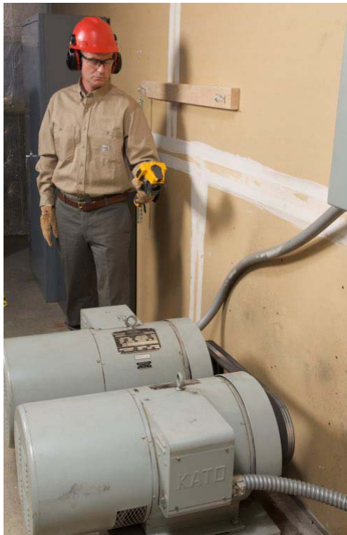
Infrared emissions from electric motors may reveal issues with bearings, drive components and overall performance.
