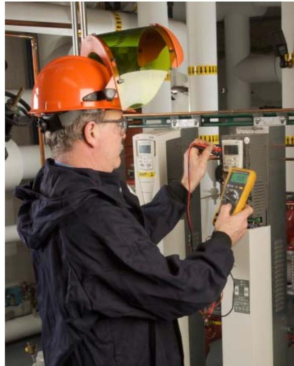
**Jim Murphy, Electrical Foreman uses the Fluke 179 DMM to look at low voltage signals in the newly installed VFD for the 40+ year old steam system.**
